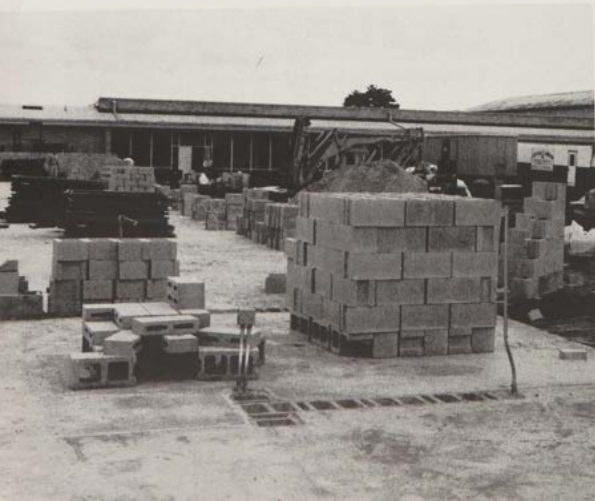
Patock Construction went to work right after ground breaking.
