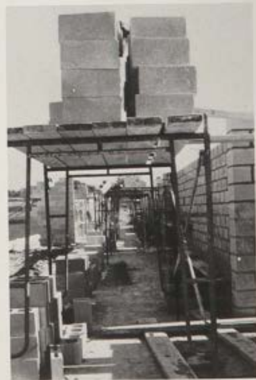
The entrance to the work site.
