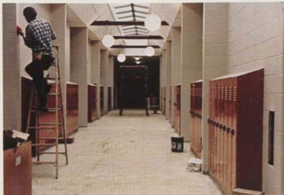
Workers add the finishing touches of the new wing.
