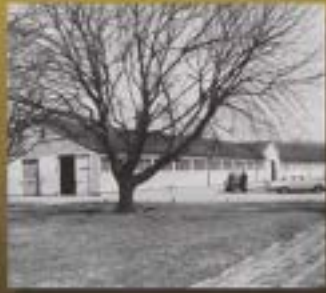
Original stable that would serve as the first temporary school building, Henderson Hall
